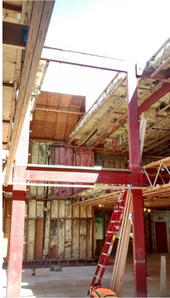
Figure 7-5 – West side of building opened up for elevator/structural work
