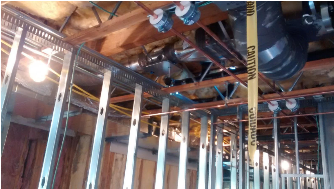
Figure 7-11 – Example of tight overhead space
